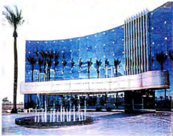
Contemporary Office Exterior
